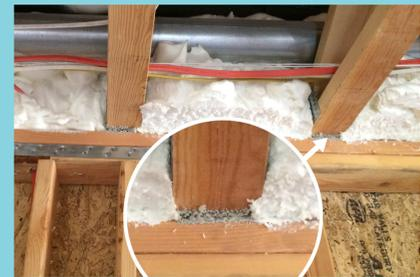
The process finds and seals leaks missed or inaccessible by manual trial-and-error methods. Results are tracked and displayed in real-time.
