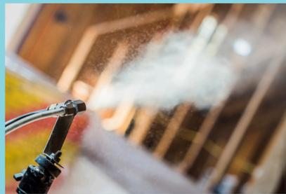
The sealing is performed by fogging a space with aerosolized sealant particles. The particles are carried to the leaks by the escaping air flow.
